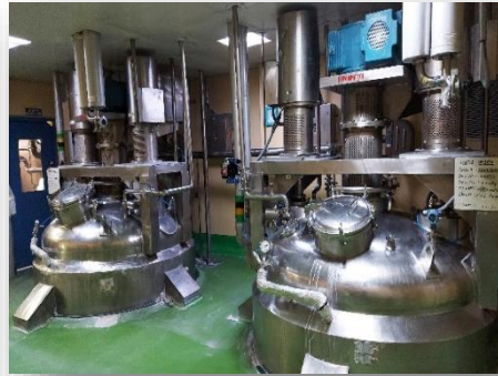
Main Mixing Tank
